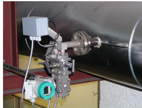
Figure 3: deltaflow for steam with integrated PT100, 3-way-manifold, mounted transmitter and connection box for cables
