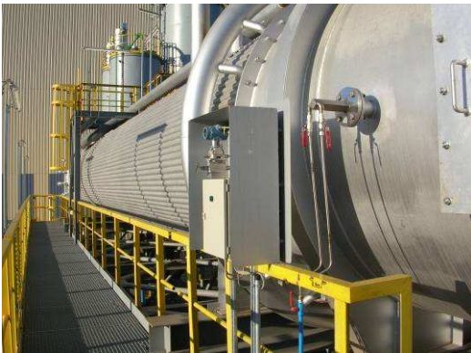
Figure 3 : deltaflow with cut ring stud, 3-way-manifold, integrated PT100 and multi variable transmitter
